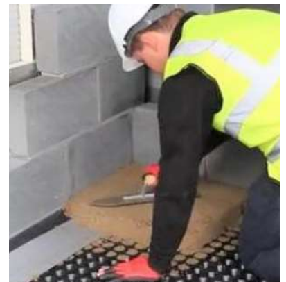
Once complete, Hydroflow HP20 is ready to receive floor screed.
