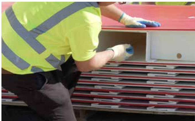
Pull down the interlocking flaps and lock into the slot provided.
