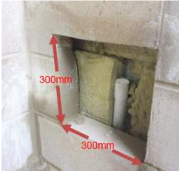
Recommended minimum access hatch size.
