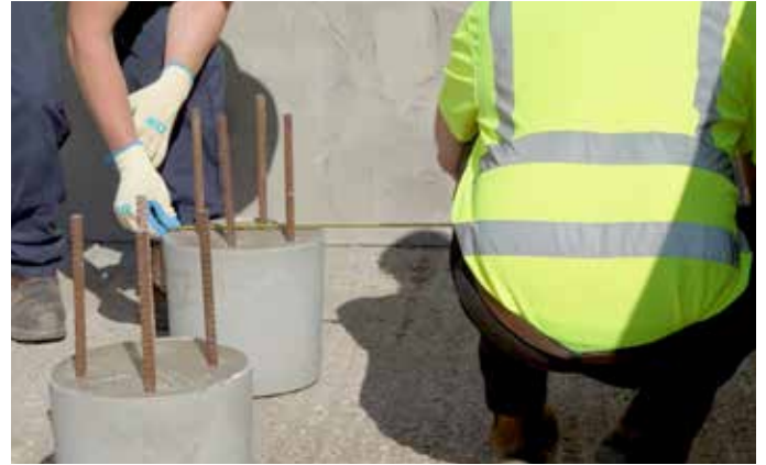
Accurately measure the pile cap diameter.
