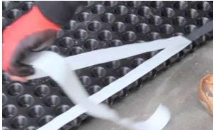
Remove release paper from Butyl tape.
