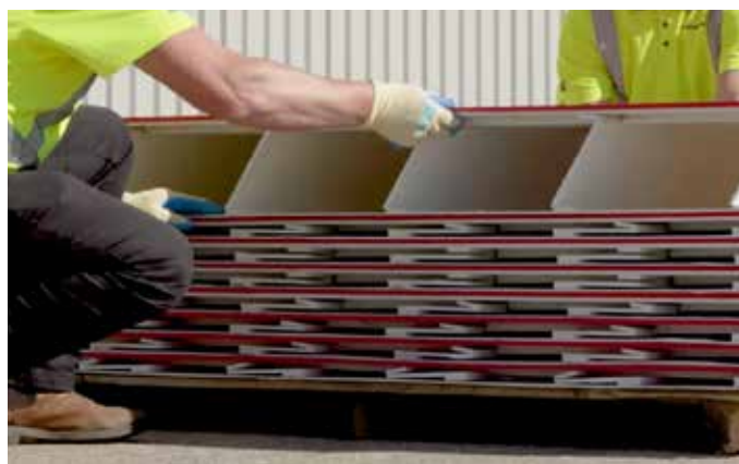
Lift top of Void-Tek panel to full height.
