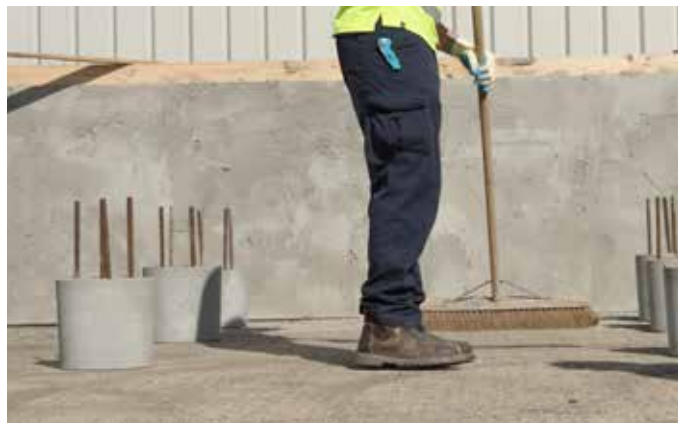
Sweep debris from concrete binding surface prior to laying Void-Tek panels.
